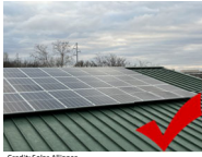
PV Array on Standing Seam Roof
